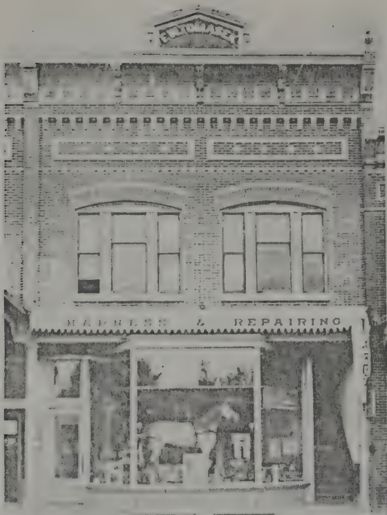
EXTERIOR, ABOVE; INTERIOR, BELOW-OF TOMASEK HARNESS SHOP
